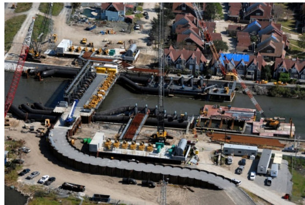
Aerial view of 17 th Street Canal during construction shows the 425-ft sheet pile-closed cell flood wall.
